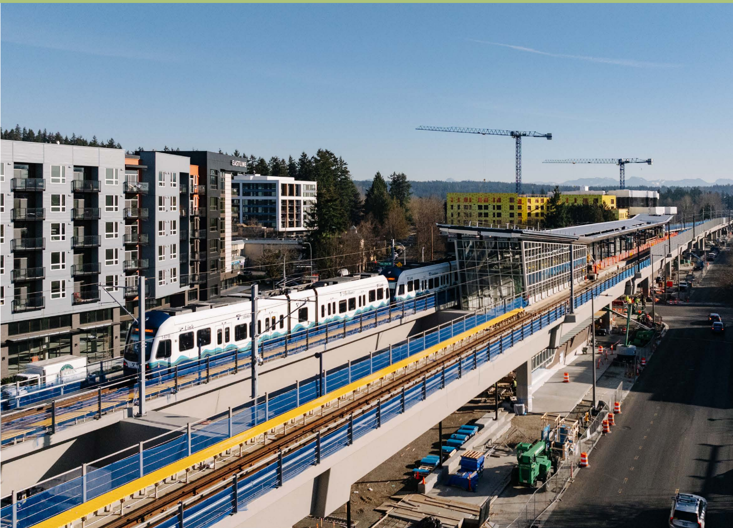
Operator qualification testing at Sound Transit’s Link Light Rail Downtown Redmond Link Extension. Photo courtesy of Sound Transit.
